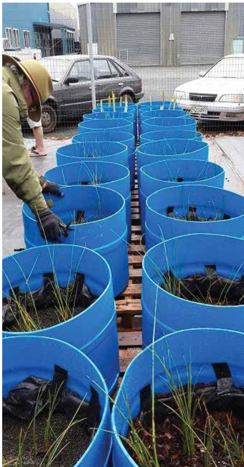
Figure 1. Establishment of the plant tolerance phase of the sludge drying bed project on site at the wastewater treatment plant in Gisborne. Wetland species have been planted into both sand and bark.
